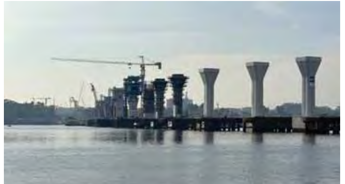
JB-Singapore RTS Link progress on track for completion
