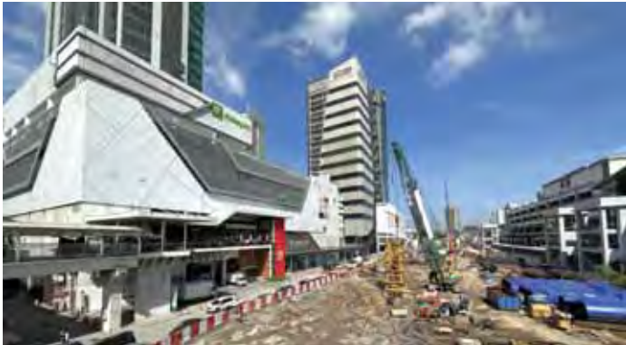
Active development underway in front of KOMTAR JBCC
